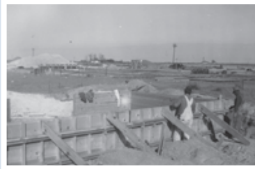
Construction of Generation Plant
