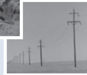
First 69 kv Line
