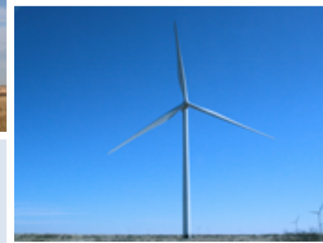
2017 Sterling Wind Farm
